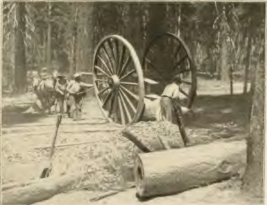
B. METHOD USED IN HAULING LOGS TO THE LOGGING RAILROAD AT SNOW, T. 40 S., R. 5 E.
